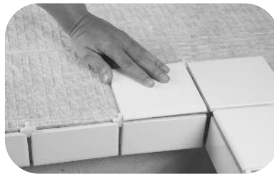
First apply tile to front of counter.
