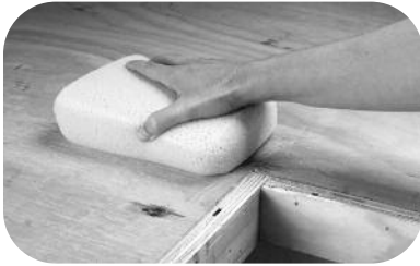
Clean dust and debris. Wipe with a damp sponge.
