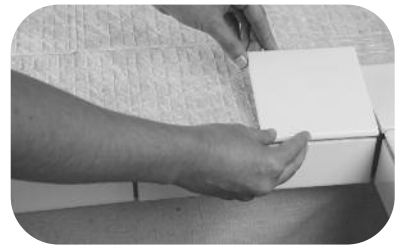
Ensure that counter tile overlaps and use spacers for a uniform grout joint.
