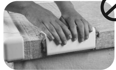
Do not apply excessive filler material as it will interfere with bond.
